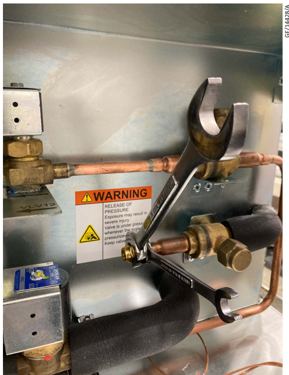
Figure 77 Install cap and flare nut on evacuation valve (MaxCool 1500 & 2200)
