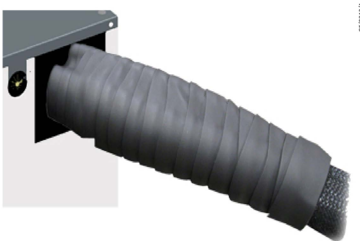
Figure 89 View of armaflex insulating tape on refrigerant line bundle on system, front access
