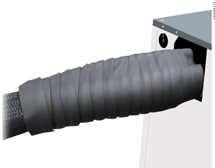
Figure 89 View of armaflex insulating tape on refrigerant line bundle on system, front access
