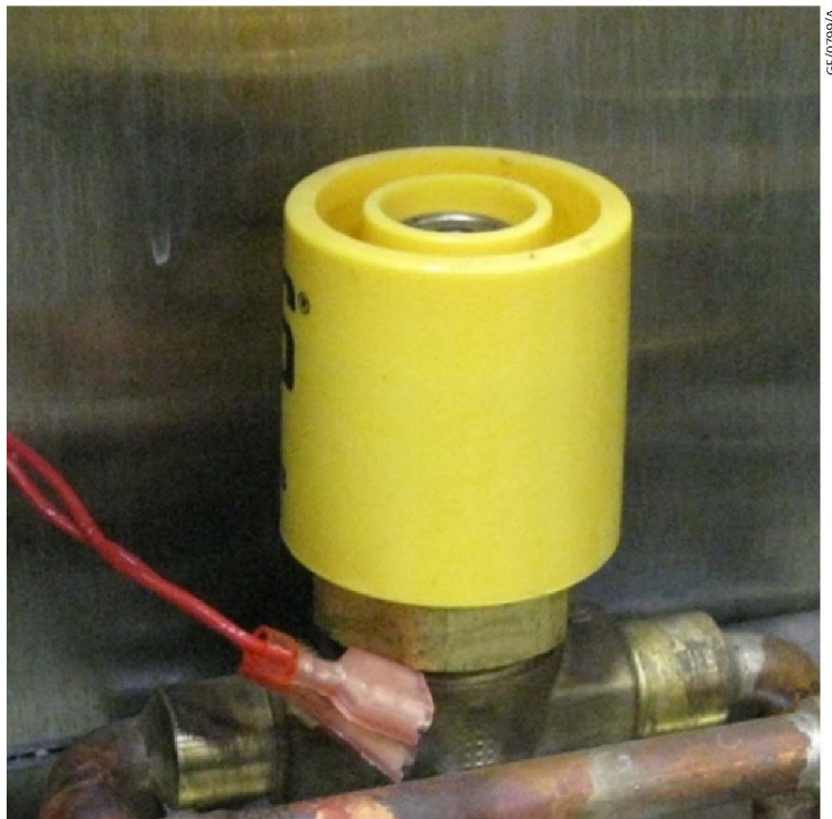
Figure 75 Coil magnet on solenoid valve
